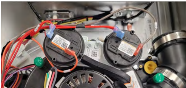
Figure 30. Pressure switch wiring
