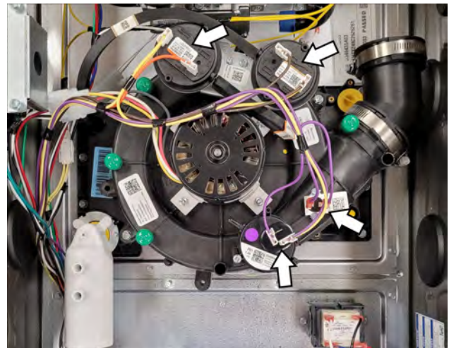
Figure 12. Inducer limit switch wiring
