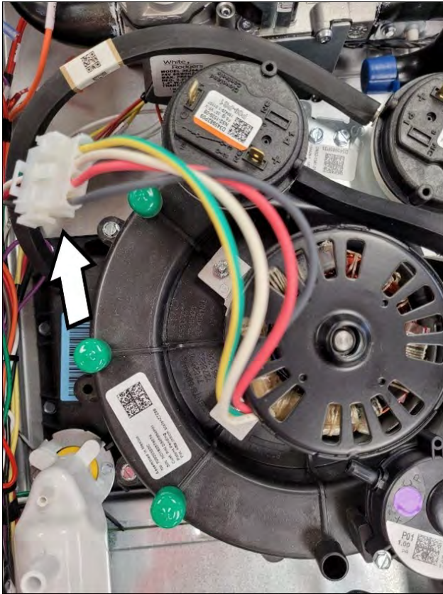
Figure 13. 4-pin inducer wire harness
