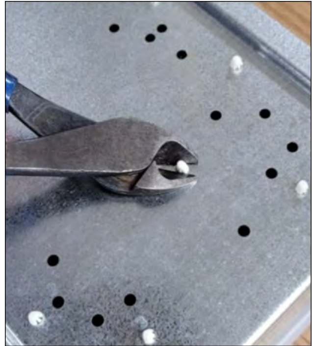
Figure 35. Remove existing IFC
