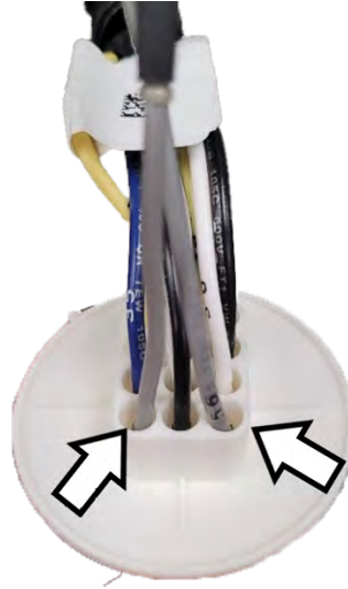
Figure 22. Install return air thermistor
