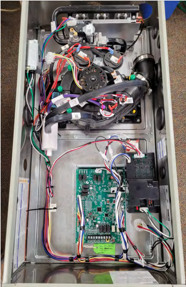
Figure 48. Complete hardware conversion
